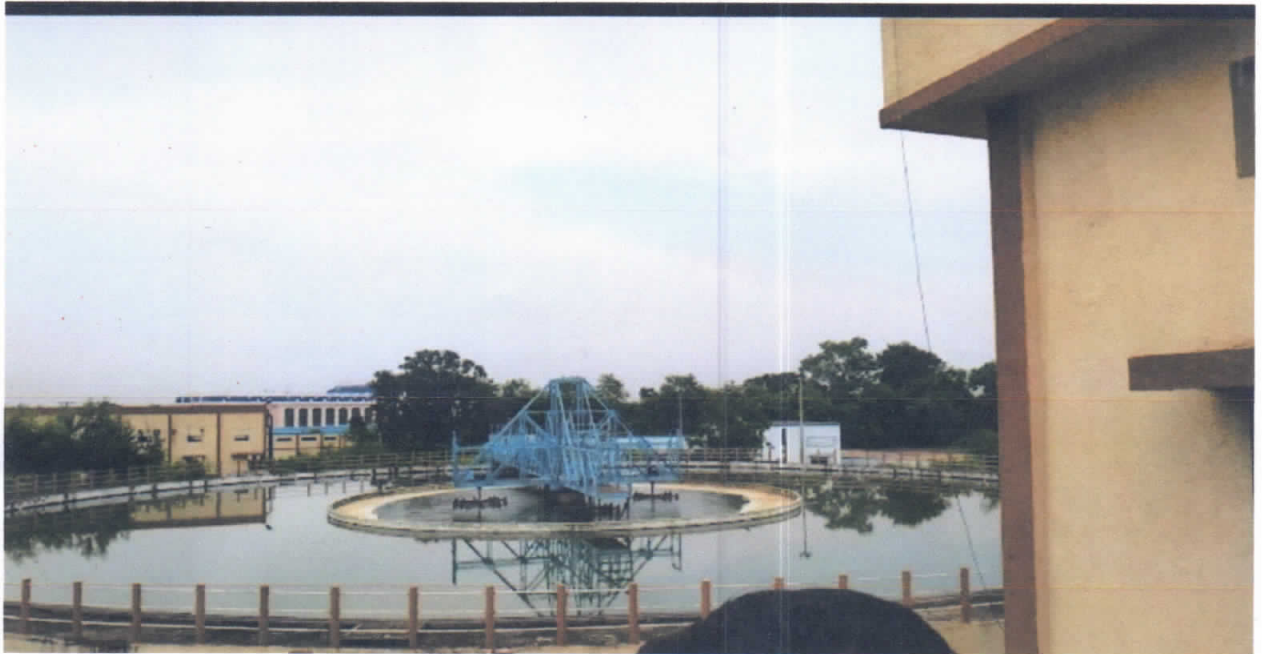
Picture of Water Treatment Plant
